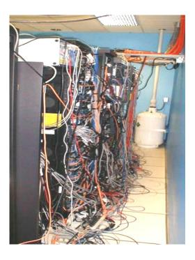
Unnecessary or unused cabling should be removed. Data cables should be cut to the right length and patch panels used where appropriate. Power to the equipment should be fed from rack-mounted PDUs with cords cut to the proper length.
