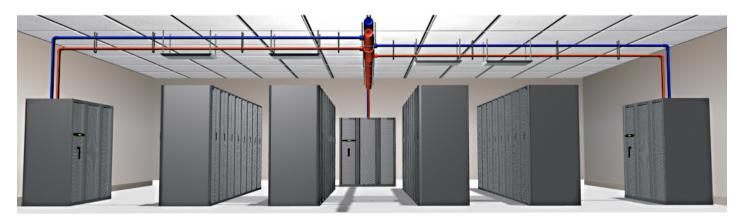
With the valves being located above the ceiling or outside the data center, balancing the cooling system is not easily done. This increases the time required for start-up and balancing of each unit. In case of leakage in an overhead installation, the repair must be performed above the equipment installed on the floor, which increases the potential for water on the floor or worst yet, the equipment.
