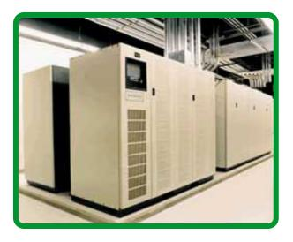
Figure 7 Centralized monolithic UPS
